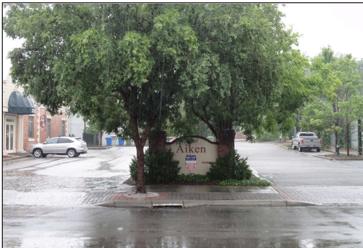
Fig. 28. This image from Aiken, SC demonstrates the ability of a porous asphalt road (right) to quickly infiltrate rain water, in comparison to standard asphalt road (left) showing puddles (Source: Calvin Sawyer, Ph.D., Clemson University).
